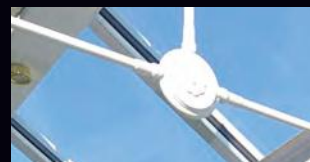
Tie bars create the classic Orangery roof space with ornate, non-structural tie bars.
