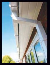
The PVCu soffits, fascias, cladding, guttering and downpipes all conform to all the relevant British Standards for durability, colourfastness, physical performance, section weight, flatness, thermal movement, fire resistance and impact resistance.
